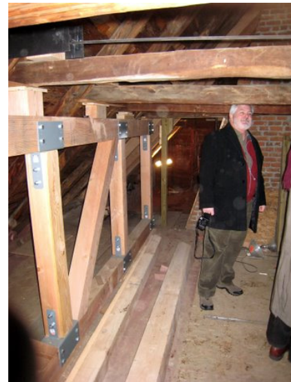
HFA Consultant Neil Larson with new north-section rafter supports
