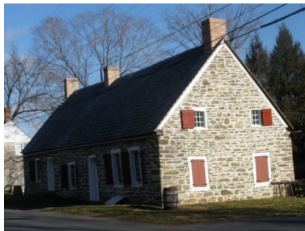
Newly installed shutters on south side of Abraham Hasbrouck House
