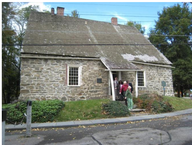
Jean Hasbrouck House showing poor condition of roof
