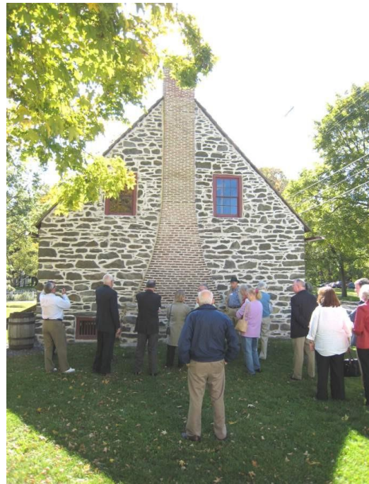
Reunion attendees view the restored north wall / chimney at the Abraham Hasbrouck House
