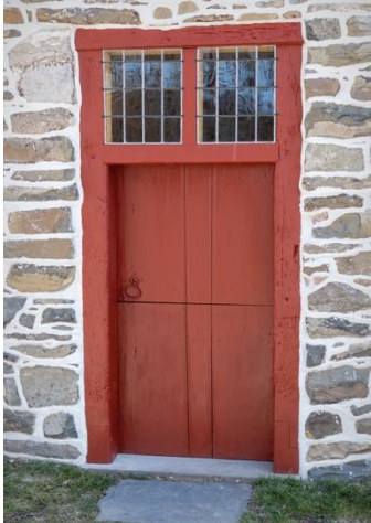
Abe House Center Room Door at ground level.
